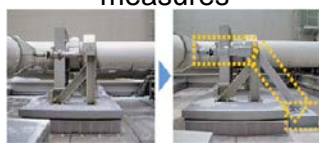
Reinforcement of piping facility
