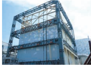
Dismantling of the building cover
