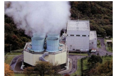
Mori Geothermal Power Plant in Hokkaido Prefecture
