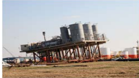
Damaged oil refining facilities
