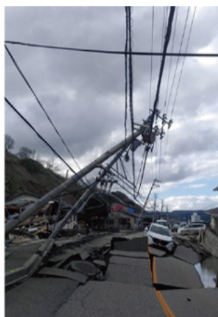
Fallen utility poles (Due to the Noto Peninsula Earthquake in January 2024) Source: Hokuriku Electric Power Transmission & Distribution Company
