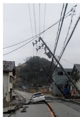
Fallen utility poles (Due to the Noto Peninsula Earthquake in January 2024) Source: Hokuriku Electric Power Transmission & Distribution Company
