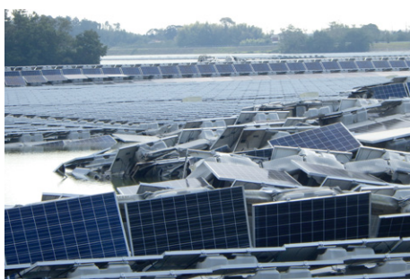
Damaged floating-type solar power generation facilities in Ichikawa City, Chiba Pref. (Due to a typhoon in September 2019)
