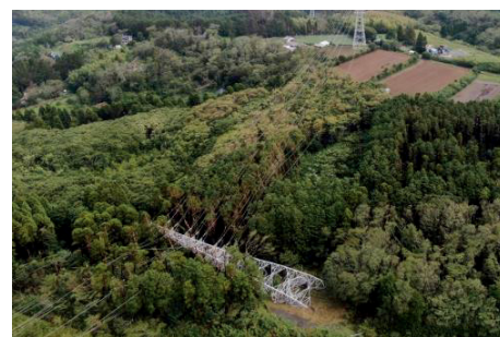
Collapsed power transmission tower in Kimitsu City, Chiba Prefecture (Due to a typhoon in September 2019)
