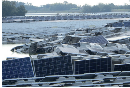
Damaged floating solar power plant in Ichihara City, Chiba Prefecture (Due to a typhoon in September 2019)
