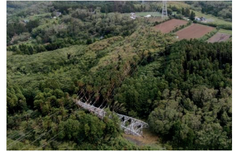
Collapsed power transmission tower in Kimitsu City, Chiba Prefecture (Due to a typhoon in September 2019)
