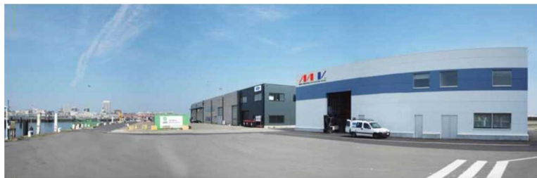
GeoSea | Parkwind | MHI Vestas
