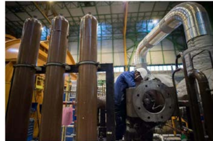
Nuclear power plant in Saint Laurent des Eaux, intervention in the machine room as part of the Grand Carénage project in October 2016
