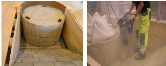
Figure 5-16. Backfilling of bevel at Äspö HRL
