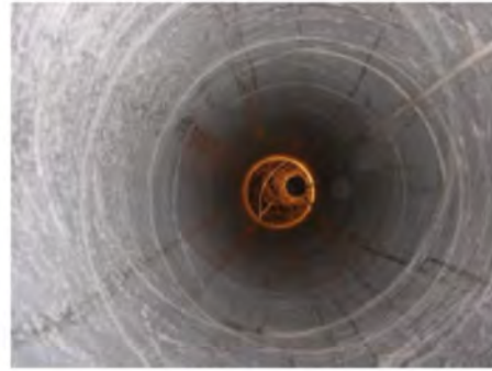
b) Gravel of fluid injection volume together with water injection tubes emerging from the inclined injection borehole
