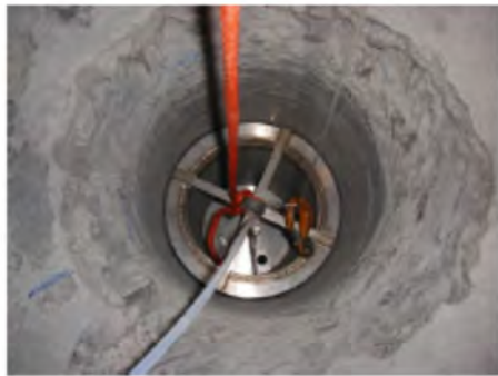
e) Packer in borehole SB2
