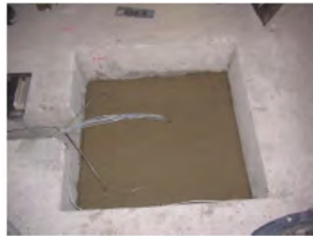
f) Grouted borehole cellar
