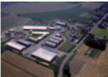
Machimura Farm Bio-gas plant (Ebetsu City, Hokkaido)
