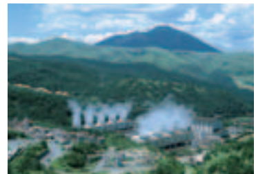
Hatchobaru Geothermal Power Plant (Kokonoe Town, Oita Prefecture)
