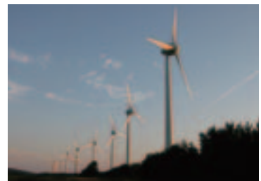
Noshiro Wind Power Plant (Noshiro City, Akita Prefecture)
